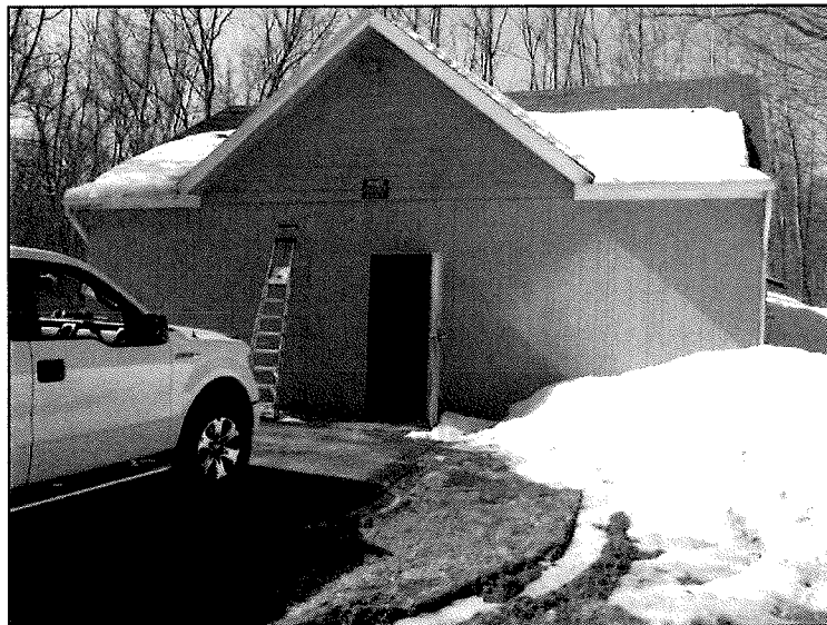
Figure 2-4 Pinebrook Treatment Facility
